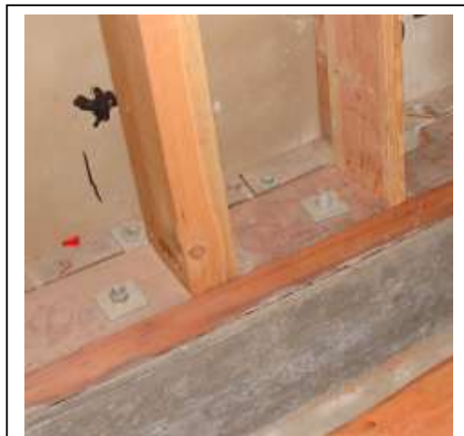
Figure 3-1 Mudsill connection to the foundation in a house under construction. This crucial connection transfers earthquake forces to the foundation.
