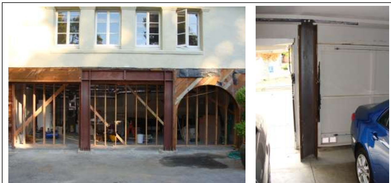
Figure 4-2 Two ways to strengthen a soft-story.
