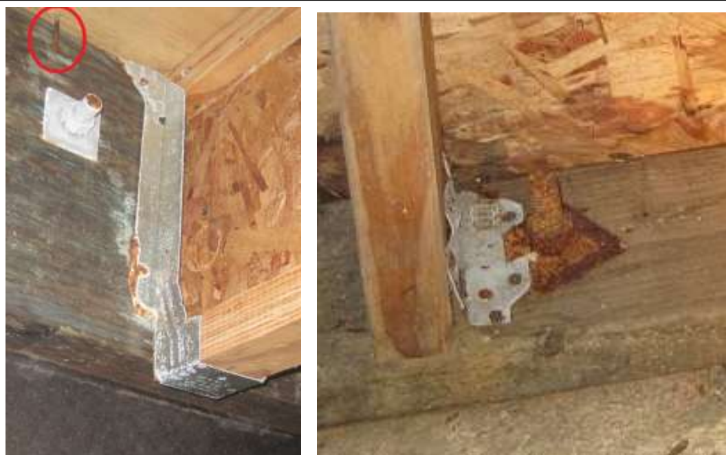
Figure 4-6 Corroding steel and galvanized steel connectors.
