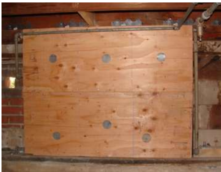
Figure 3-7 Plywood bracing panels nailed along all edges. Note the horizontal joint with nailing above and below the joint. The six holes provide ventilation to help prevent moisture build-up and associated damage
