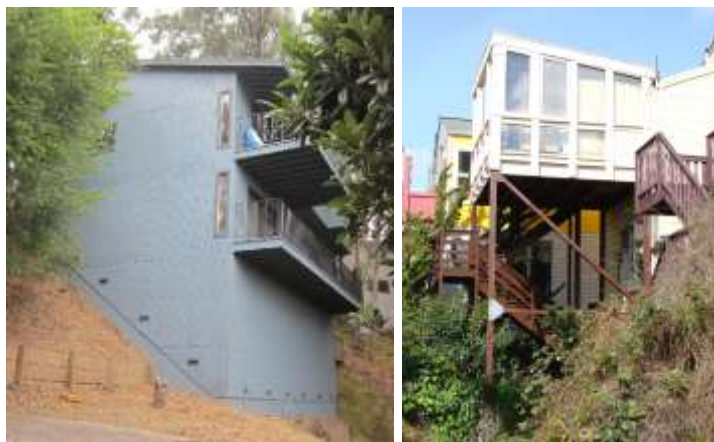
Figure 5-1 Hillside homes require special consideration; plywood shear walls perform badly in sloping walls as found in the house shown above left. Homes on steep sites can be very dangerous in quakes.
