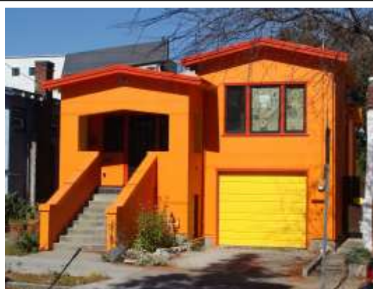
Figure 2-1 Typical house with cripple walls.
