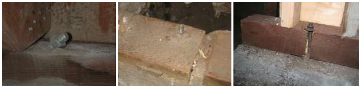
Figure 3-6 These photos show several examples of bad anchor bolt installations: Left: Retrofit bolt installed at an angle; Center: Bolt that is too small, installed without a proper washer and too close to the end of the mudsill; Right: Mudsill slotted to install in the course of repairing decay or pest damage. • PH. Matt. PR
