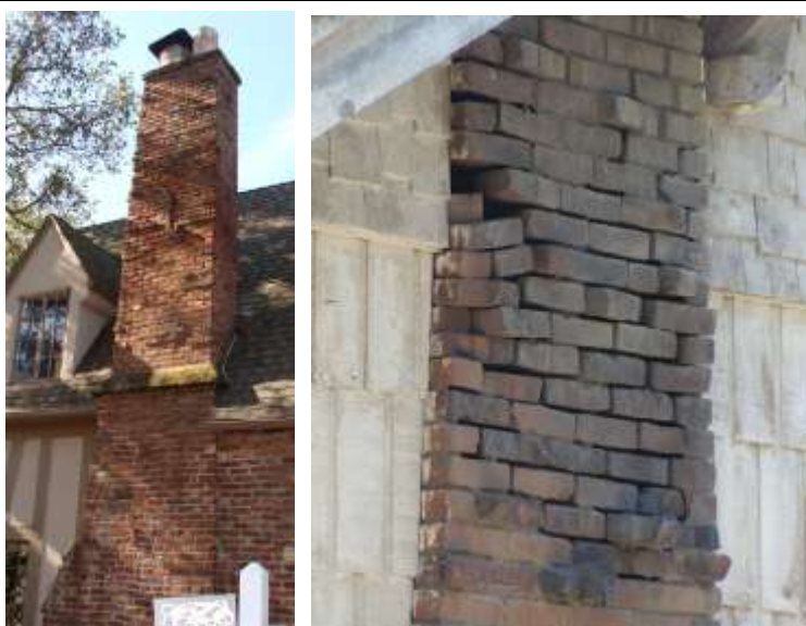
Figure 4-8 Chimneys are hazardous even when they are in good condition. Slamming the front door could cause the disintegrating chimney shown at right to collapse.
