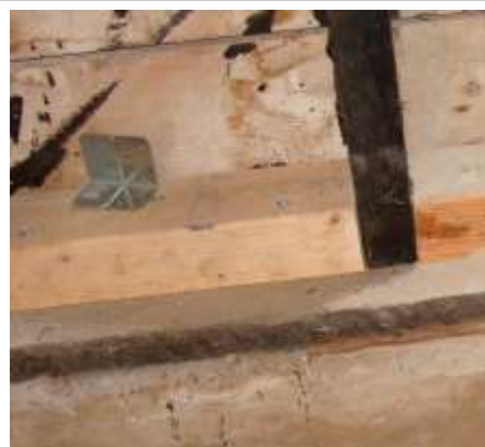
Figure 3-8 Mudsill blocks connected with structural screws.
