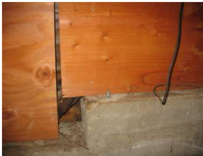
Figure 3-11 Plywood must be nailed to framing along each panel edge. TM—Max Cullen/W
