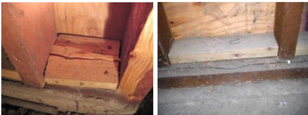
Figure 3-12 Mudsill block problems: Left—Split block; Right—lack of visible connection from block to mudsill. TM—RPaul Rude
