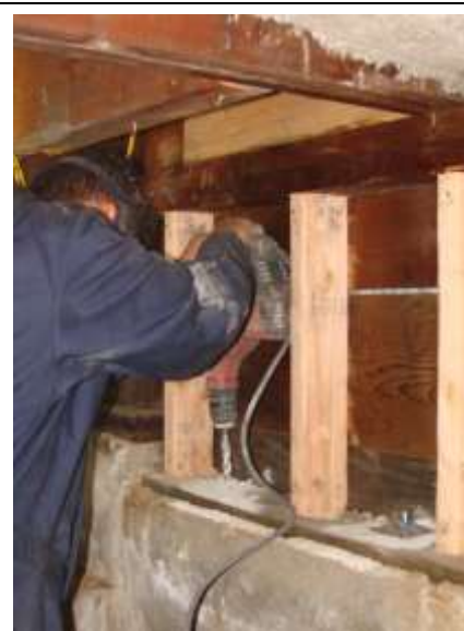
Figure 3-3 Retrofit bolt installation at a cripple wall.
