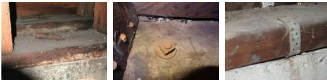
Figure 3-2 Mudsill connections used in the past. From left to right: Steel rod, pin, or bolt bent down over mudsill; bolt with standard round washer and nut; proprietary sheet-metal strap embedded in concrete and wrapped around and nailed to mudsill.
