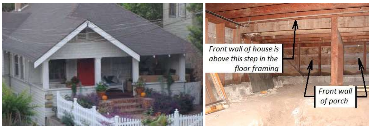
Figure 4-3 Front wall without foundation. The photo at right was taken in the crawlspace looking toward the front of the house. The foundation follows the porch outline; there is no foundation below the front wall of the house.
